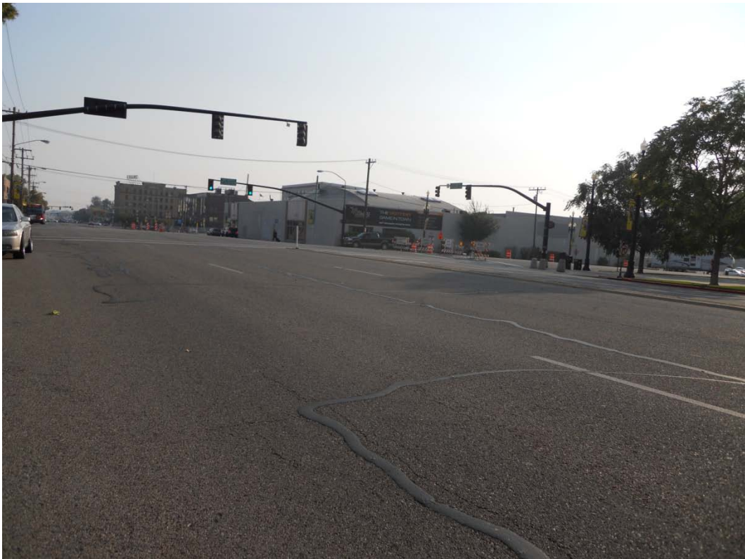
300 West 100 South intersection (looking southwest)
